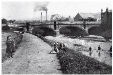
By the early 19th century there is recorded evidence of a narrow bridge over the River Irvine. In 1839 a three span suspension bridge known as Galston Bridge or The Muckle Bridge was constructed replacing a ford, built from sandstone with three arches which helps give it strength. At this time it was seen as a major structure and a feat of engineering. Stone from the Gauchalland Quarry was used.
